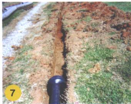
7 CPP No-Rock Septic pipes allow for narrow trenches that offer a closer OC spacing, which requires a reduced land area foot print compared to conventional 3-foot wide trenches.
