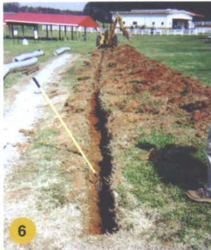
6 Trenching complete, and ready for Side-Wall rake prep sequence.
