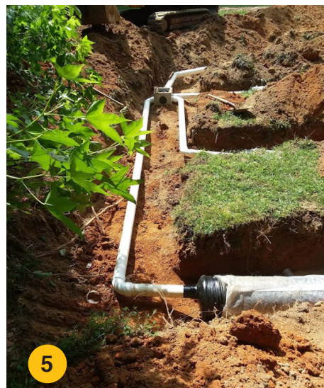
5 D-Box connections to 6FT OC trench spacing.
