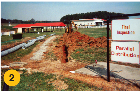
2 Protective plastic bags removed just prior to trench placement.
