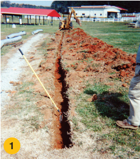
1 Trenching complete, and ready for Side-Wall rake prep sequence. If needed.
