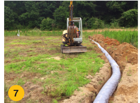
7 Pipe flex follows site contour.
