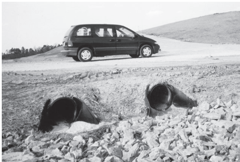
CPP HDPE Flared Ends in combination with Cap Stone at the water discharge end stabilizes erosion before and after site work seeding and paving.
