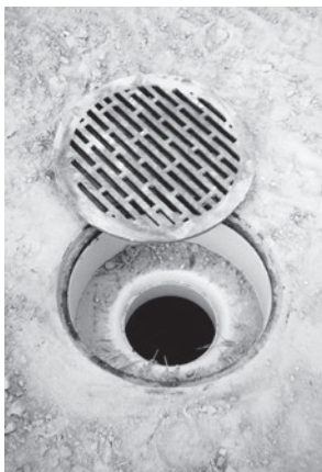
Inlet Drain frame and grate ready for paving and/or seeding.
