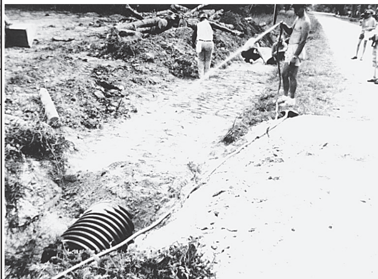
Stiff Soil under, around and on top
